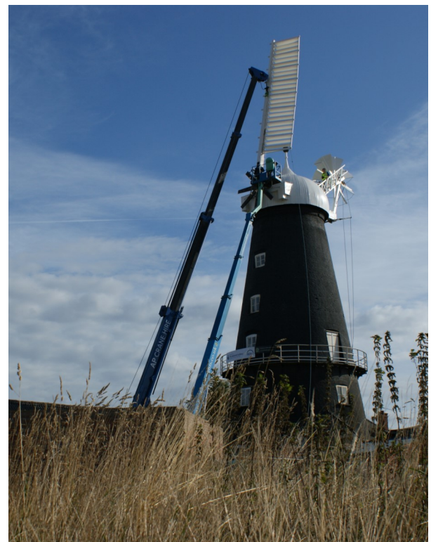
The first of the new sails being fitted to the mill tower
